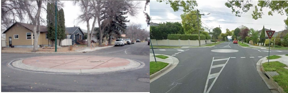
Figure 2: Examples of mini roundabouts. Note that these can be constructed without necessarily needing to acquire land at the four corners of the intersection
