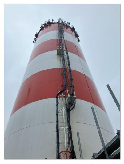
The cables have been relocated to new cables trays located on either side of the new safety ladder. The antennas' mounting system is now under review and could force the project to be overbudget if important upgrades are required.
